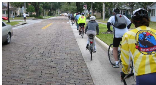
The model for brick streets with smooth concrete bike lanes on Livingston Street is recommended for use on other brick roadways having sufficient width or those that may be converted to brick.
