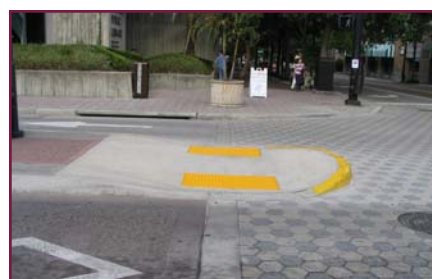
(top) Two curb ramps per corner provide the best accommodation for all pedestrians (Photo: Dan Burden).
