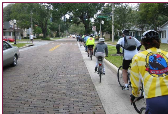
As part of the City's effort to become more bicycle friendly, Livingston Street in Downtown Orlando was converted from a three-lane facility (left image) to a two-lane brick street with concrete bike lanes (right image).
