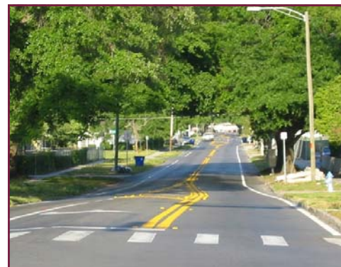
The shoulder on Washington Street, shown here between Westmoreland Drive and Parramore Avenue, is not striped correctly for bicycle traffic and disappears at major intersections.
