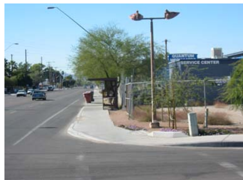
Figure 5. A new segment of ADA-accessible sidewalk as part of a major roadway improvement project.
