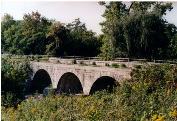
The Flatstone Creek Aqueduct, built in 1898, is a typical canal feature associated with the trail.
